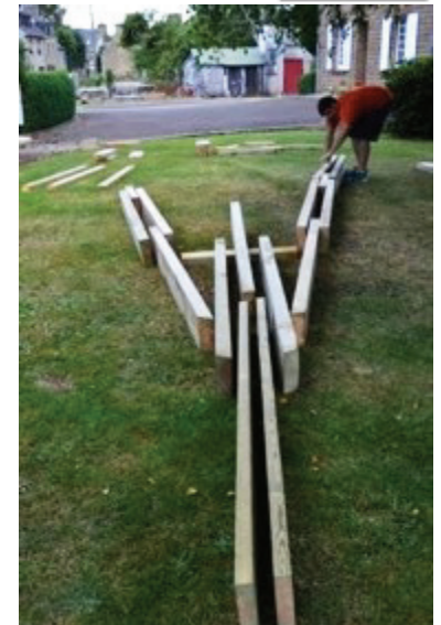
Assembling the Tower
