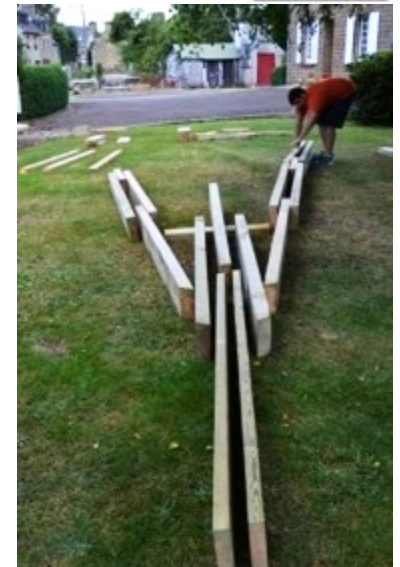
Assembling the Tower
